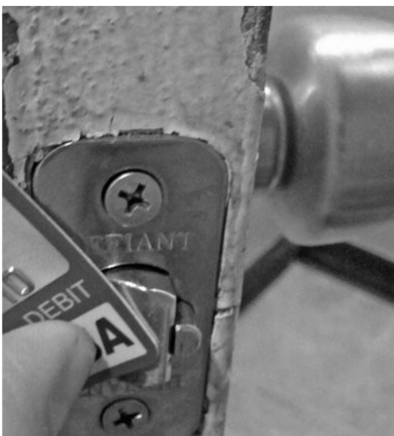
Figure 9-13 Shimming lock plunger with credit card
