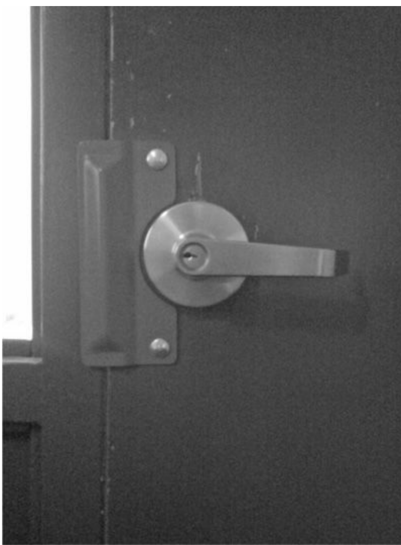
Figure 9-14 Shim guard blocking access to plunger
