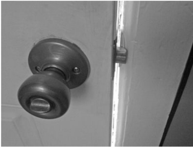
Figure 9-3 Door plunger mechanism and door strike plate
