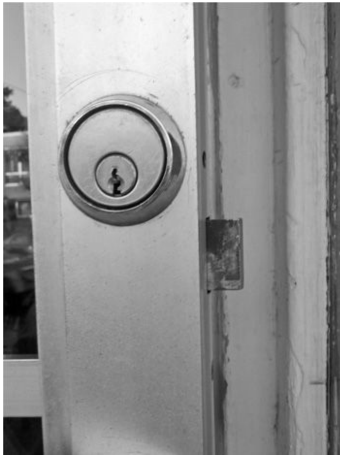
Figure 9-4 Deadbolt-type straight plunger
