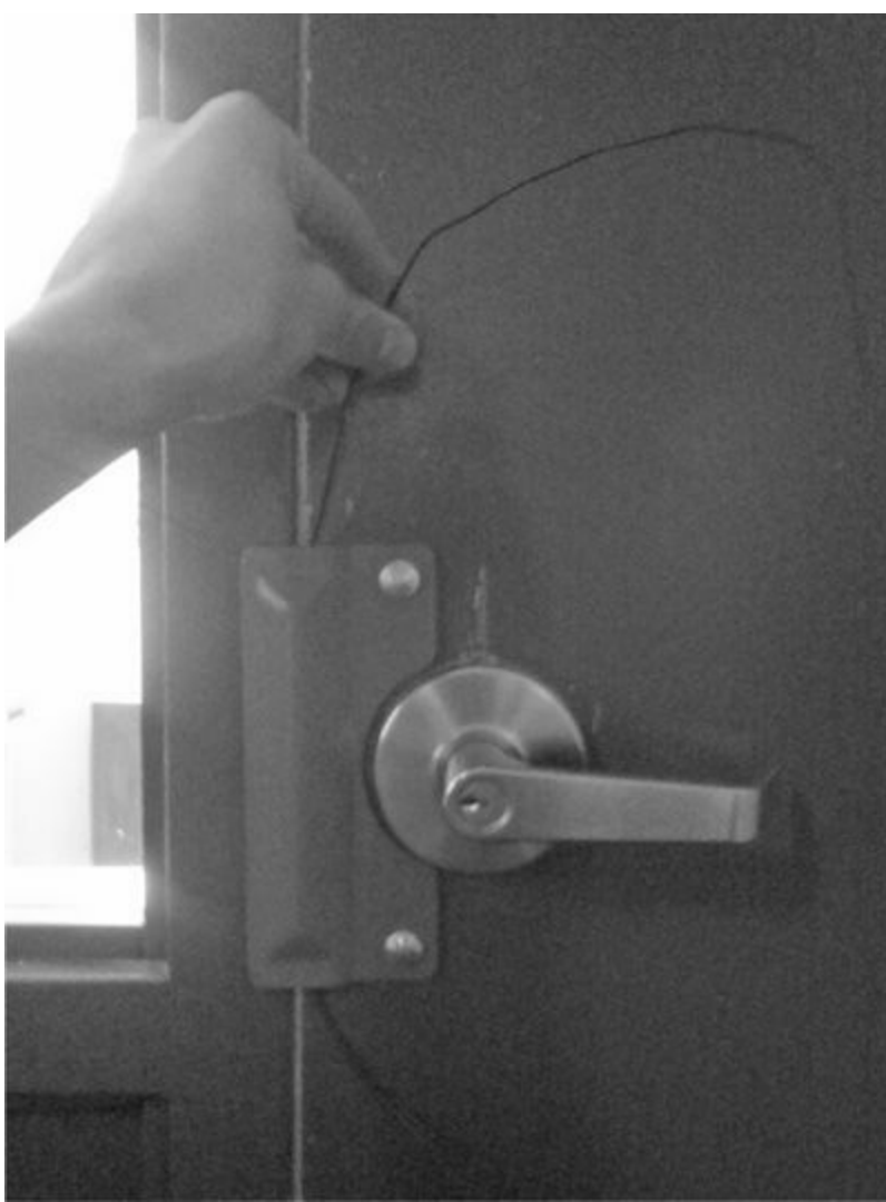
Figure 9-15 Bypassing shim guard with thin cable
